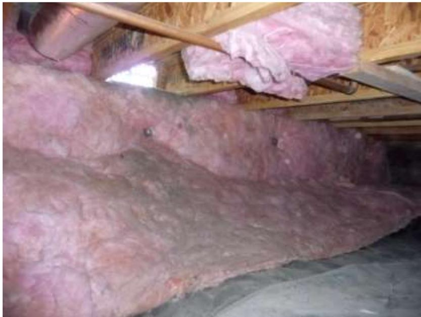
In this picture, to the left, you can see how close the main 1" domestic water line is installed to my "open" crawl space vent grille opening (about 3+ feet). Apparently a kindly, and observant, insulation worker - realizing the poor placement of the main 1" domestic water line - took it upon himself to hang a little insulation over the piping in hopes of giving it a little protection.
